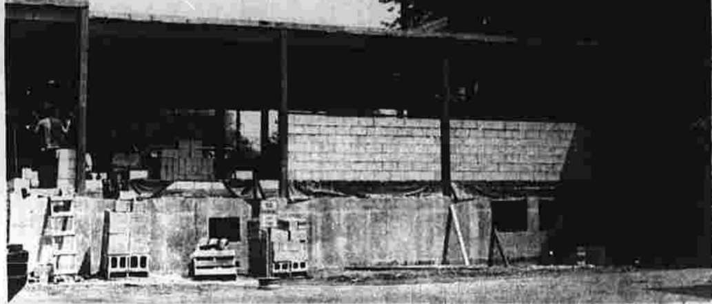
Walls rise at police station addition
